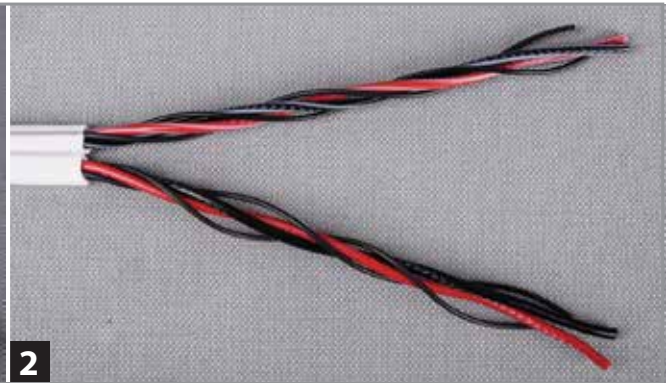
2. Remove the PVC jacket.
